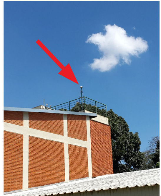
FIGURE 20 GNSS antenna of EESC0 mountpoint (photograph taken by author on 6 April 2018)
